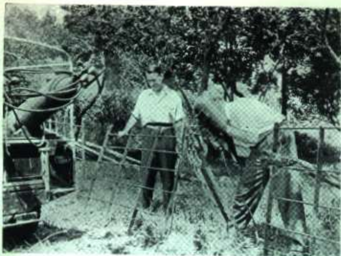
Repairing Fences — Welding
